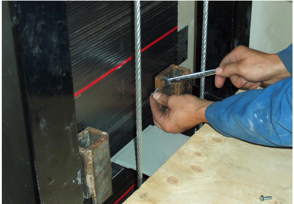
Figure 12. Removing the counterweight hangars.
